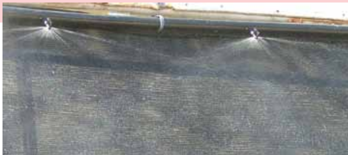
Modular half-circle sprayer 100 l/h mounted every 1.0 m
